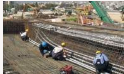
Fig.2 Recommended Ducts Arrangement
