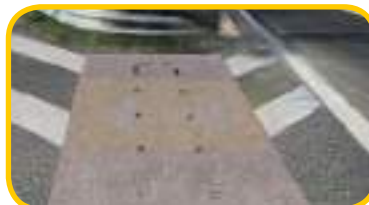
Precast Concrete Basement
