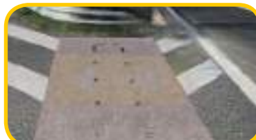
Precast Concrete Basement
