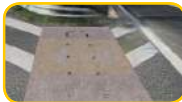
Precast Concrete Basement
