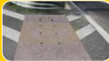
Precasted concrete basement
